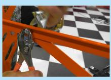
8. Then begin bolting the X cross braces starting with the center bolt and nut and then bolt it to the horizontal beams top and bottom
